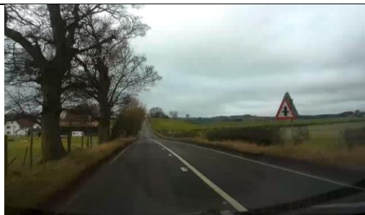
Photo 7- Example of location where enhancement of the warning sign, with a supplementary distance plate may be beneficial.
