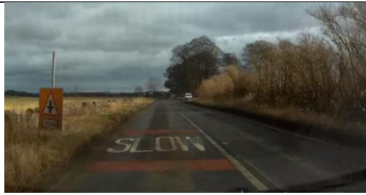
Photo 37 – Yellow back crossroads warning sign has slipped on existing post.
