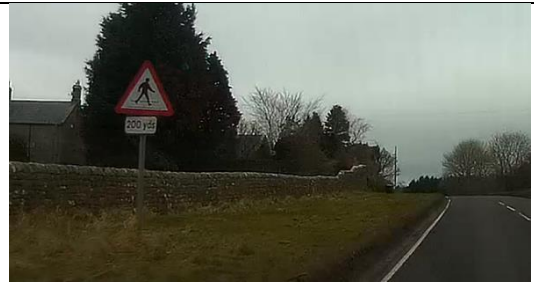
Photo 22 – Incorrect signage in place for a location where pedestrians cross.
