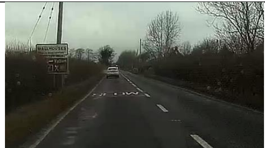
Photo 16 - Example of advanced direction obscured by vegetation.
