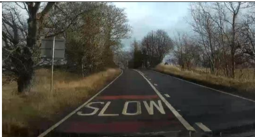
Photo 35 - Warning sign has been twisted to face wrong direction
