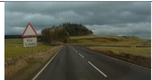
Photo 26 – Badly worn double bend warning sign. Sign and supplementary plate could be enhanced on yellow backing board
