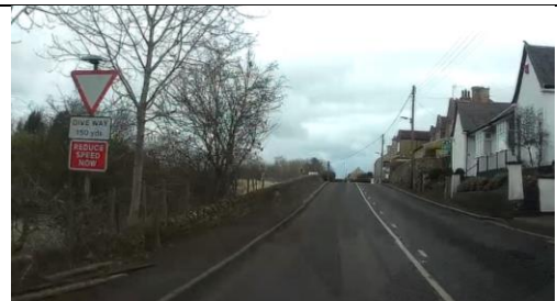
Photo 42 – Advance junction warning sign could be enhanced and provided with SLOW markings and red strips.
