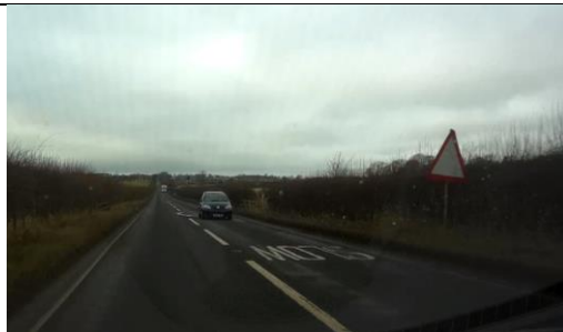
Photo 15 – Warning sign face is badly worn and requires replacement and sign is twisted to face in the wrong direction.
