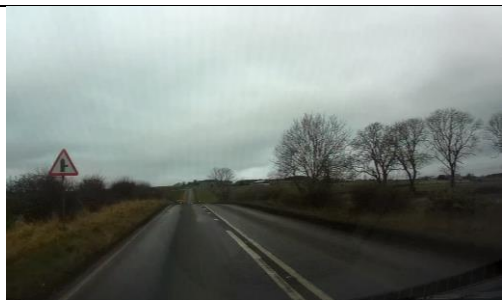
Photo 11 – Ensure termination of double white line system is located correctly, opportunity to enhance junction warning sign and provide SLOW roadmarkings and red surface strips.
