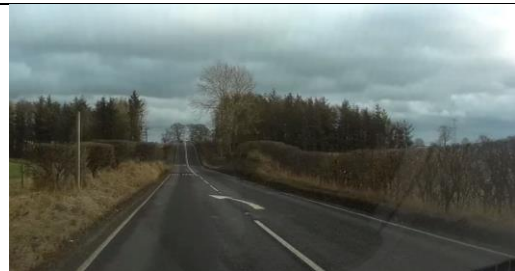
Photo 24 – Missing warning sign (vacant post) in advance of a section of road with non standard vertical and horizontal alignment.
