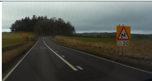
Photo 23 - Example of use of double banked double bend warning signs with advisory speed limit supplementary plate.
