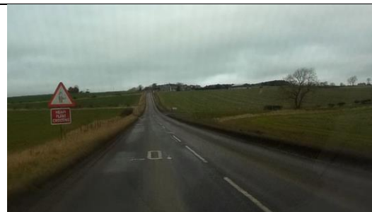
Photo 12 - Example of worn sign and SLOW road markings which can be improved.
