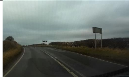
Photo 6- Example of location where enhanced chevron signing on bend may be beneficial along with road marking/stud refreshment.
