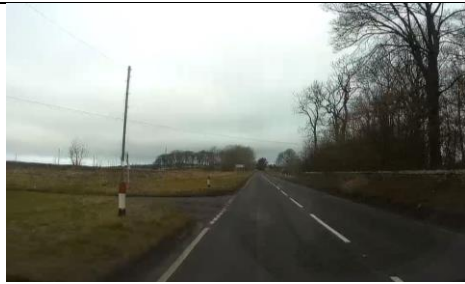
Photo 21 - Example of use of marker posts to highlight presence of minor side road junction.
