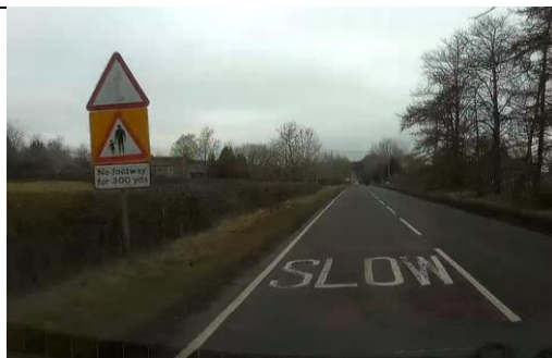
Photo 17 - Warning sign face is badly worn and requires replacement
