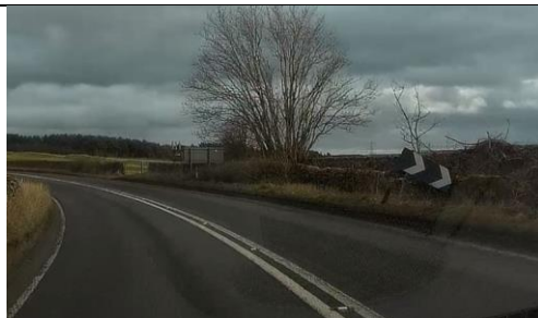
Photo 27 – Chevron sign has been dislodged and is facing the wrong way – should be directing traffic left around the bend.
