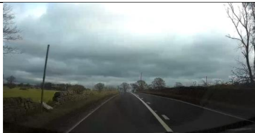
Photo 25 - Missing warning sign (vacant post).
