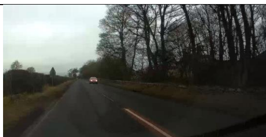
Photo 19 – Example worn set of road markings/studs alongside other markings which have been refreshed more recently.
